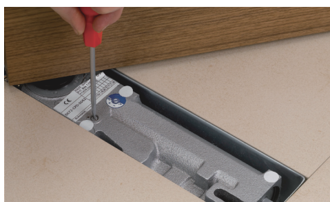
Floor spring adjustments
