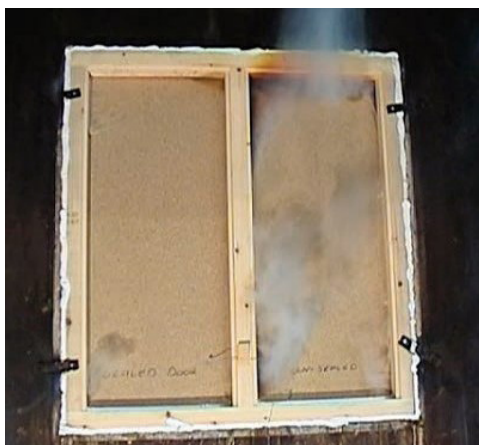
Without smoke seals, smoke passes around fire doors in the early stages of a fire - note the unsealed right hand door
