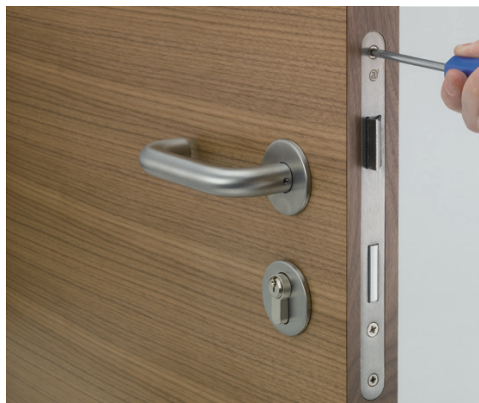
Lock tightening
