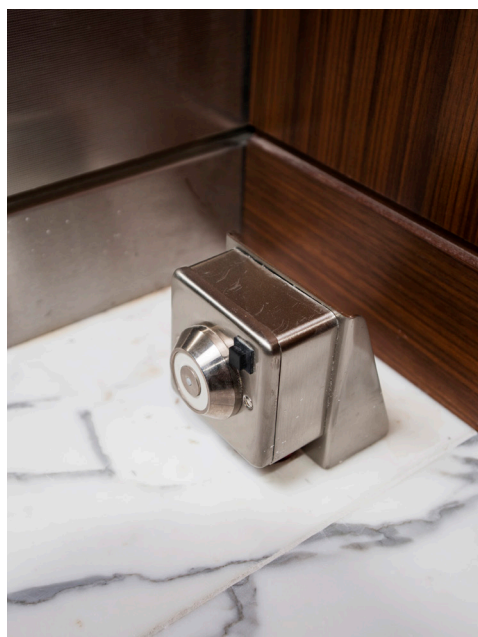
Separate hold open electro-magnet
