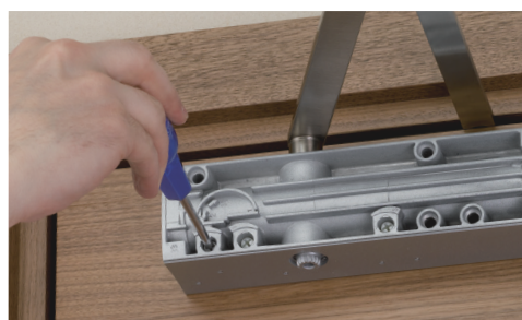
Overhead door closer adjustments
